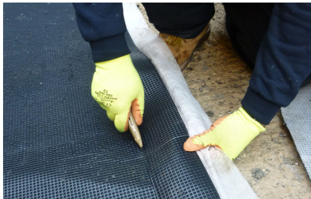
Fig. 6: Cut Deckdrain to length using a safety knife
