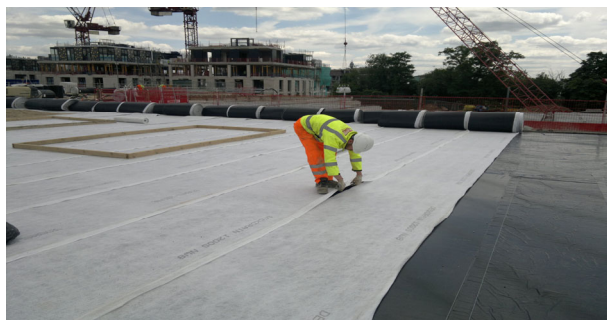
Fig. 6: Cut Deckdrain to length using a safety knife
