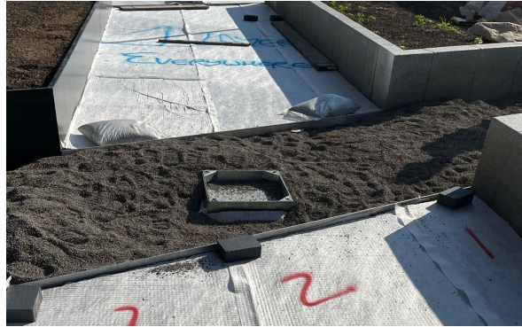
Fig. 12: Non-load bearing walls and planters can be built off Deckdrain if a suitable concrete footing is cast.
