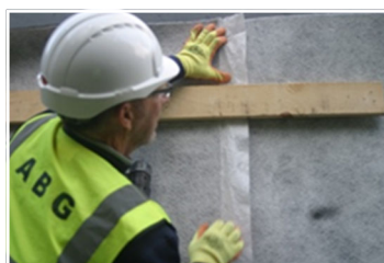
Fig 2: Hang first and second panels. Ensuring overlaps in place
