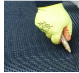
Fig 1: Roll out and cut Deckdrain with safety knife
