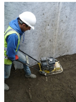
Fig 10: Shovel soil to level and use vibrating plate next to Deckdrain
