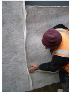
Fig 8: Place second layer and ensure flaps overlap horizontally and vertically
