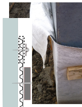
Fig 11: 300 mm textile tucked behind Deckdrain and overlapped
