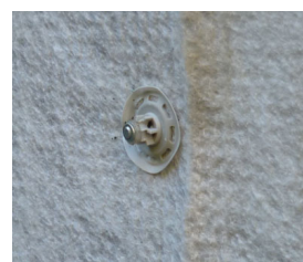
Fig 3: Fasten midwall with nail and plastic washer
