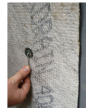
Fig 4: Alternative fixing method using Abfix stickpins. Remove protective release paper and press pin firmly to wall. Surfaces should be clean and dry, free of dust, grease, oil and any other loose matter. Impale Deckdrain over the pin, secure in place with washer then flatten pin.
