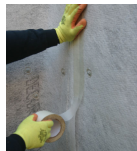
Fig 6: Seal flaps with ABG jointing tape
