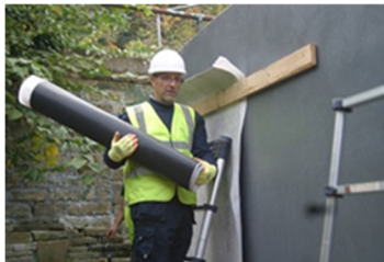
Fig 1: Roll out and cut Deckdrain with safety knife
