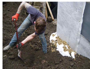
Fig 10: Shovel soil to level and use vibrating plate next to Deckdrain
