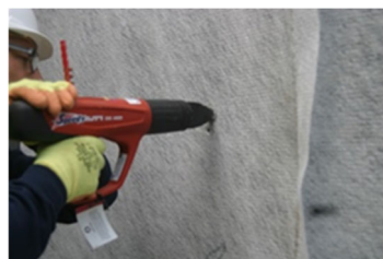
Fig 3: Fasten midwall with nail and plastic washer
