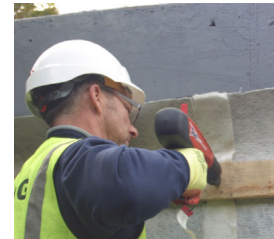
Fig 1: Roll out and cut Deckdrain with safety knife
