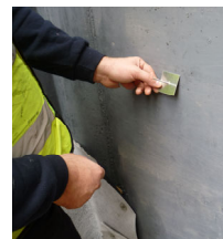
Fig 4: Alternative fixing method using Abfix stickpins. Remove protective release paper and press pin firmly to wall. Surfaces should be clean and dry, free of dust, grease, oil and any other loose matter. Impale Deckdrain over the pin, secure in place with washer then flatten pin.
