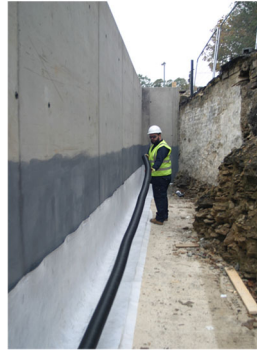
Fig 7: Roll out and cut Deckdrain with sharp knife
