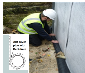
Fig 5: Wrap pipe to just cover pipe and weight down
