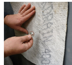
Fig 4: Alternative fixing method using Abfix stickpins. Remove protective release paper and press pin firmly to wall. Surfaces should be clean and dry, free of dust, grease, oil and any other loose matter. Impale Deckdrain over the pin, secure in place with washer then flatten pin.
