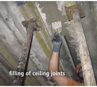
liquid-tight repair at gas stations
