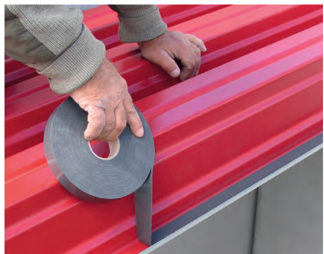
Installation example: ISO-ZELL FIX-TAPE
