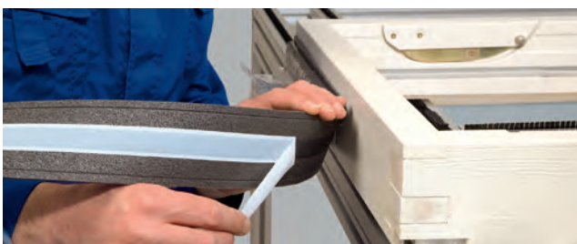
Installation example (1-BT): Fitting wooden windows
