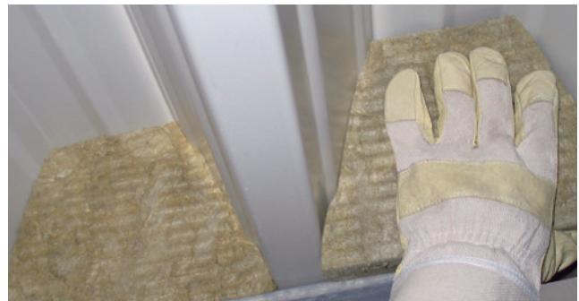
Installation example: ISO-PROFIL FILLER PIECES
