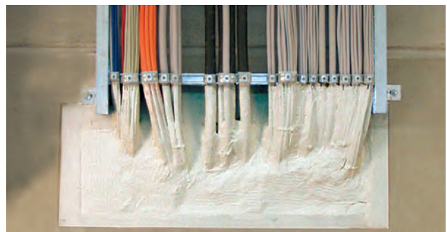
Installation example: ISO-FLAME BRICK S 90
