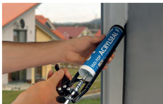
Installation example: ISO-TOP ACRYLSEAL F
