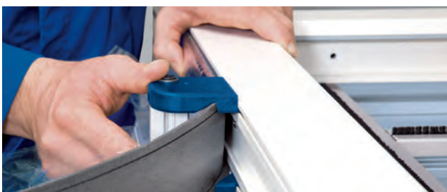
Installation example (CB): Fitting PVC windows
