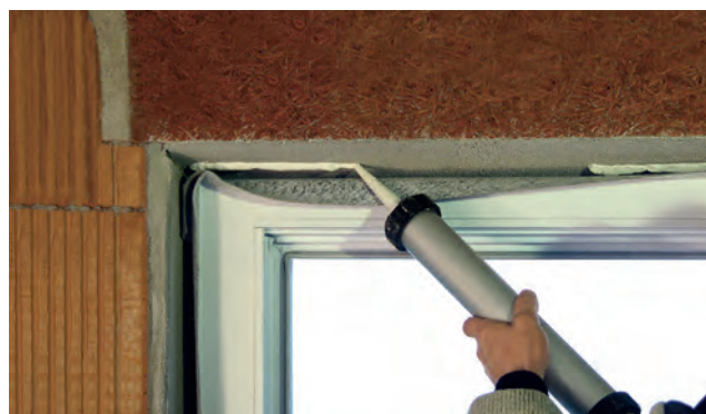
Installation example: ISO-TOP FLEX-ADHESIVE SP
