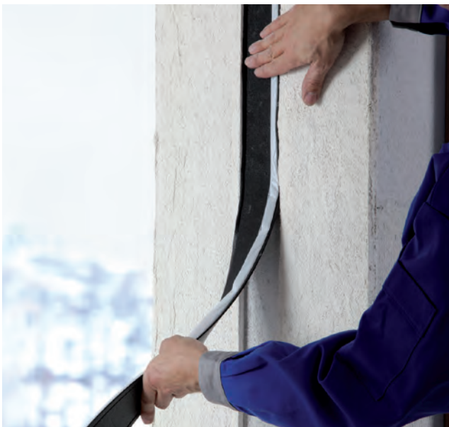
Installation example: ISO-BLOCO RENO
